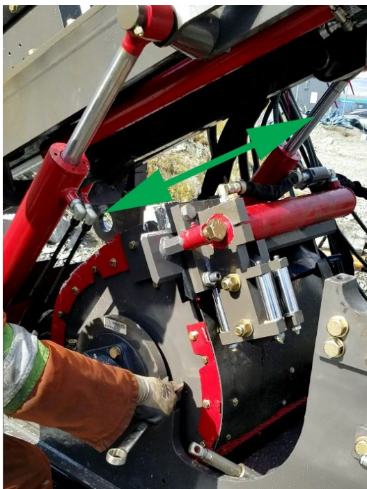
Figure 44 Anchor bolt aligns with the mast.
